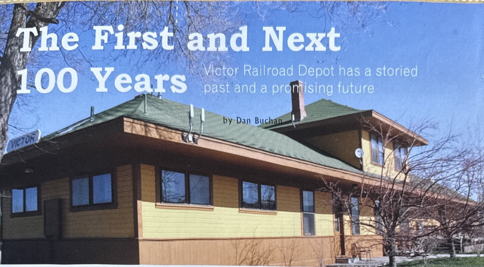
The Victor Depot as it appears today (above) and a schematic of what the site will look like after the depot revitalization and addition of the scenic byway interpretive center.
